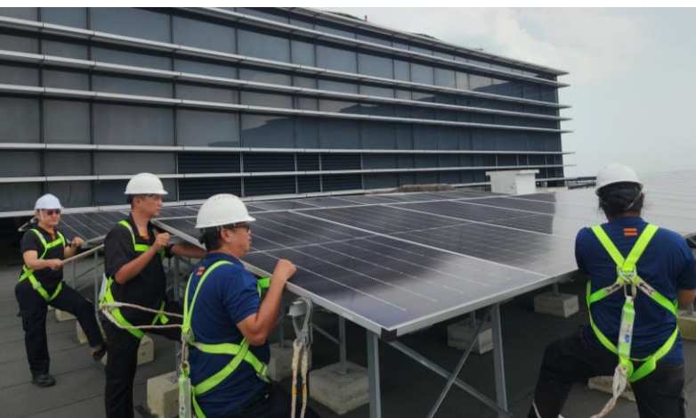
Solar panels being installed at MBC, Singapore
